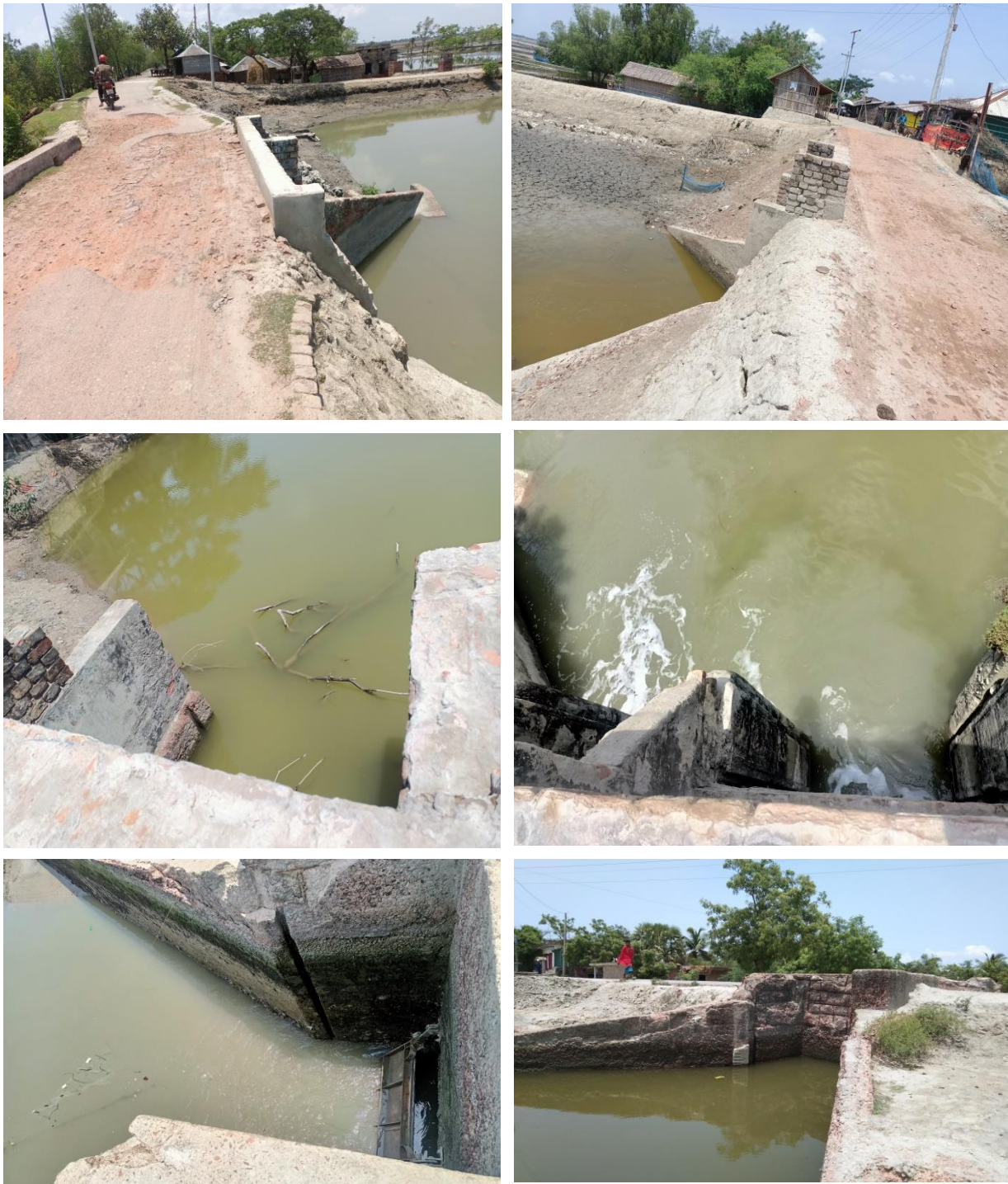
Figure 2-12: Existing conditions of the sluice gates in 10/12 polder
