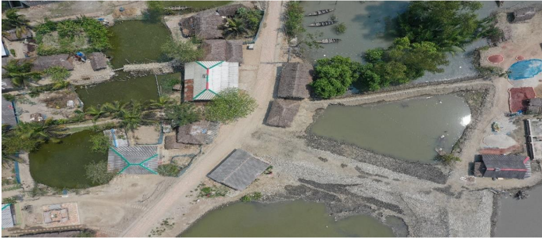
Figure 2-6: Existing Condition of Polder 10_1
