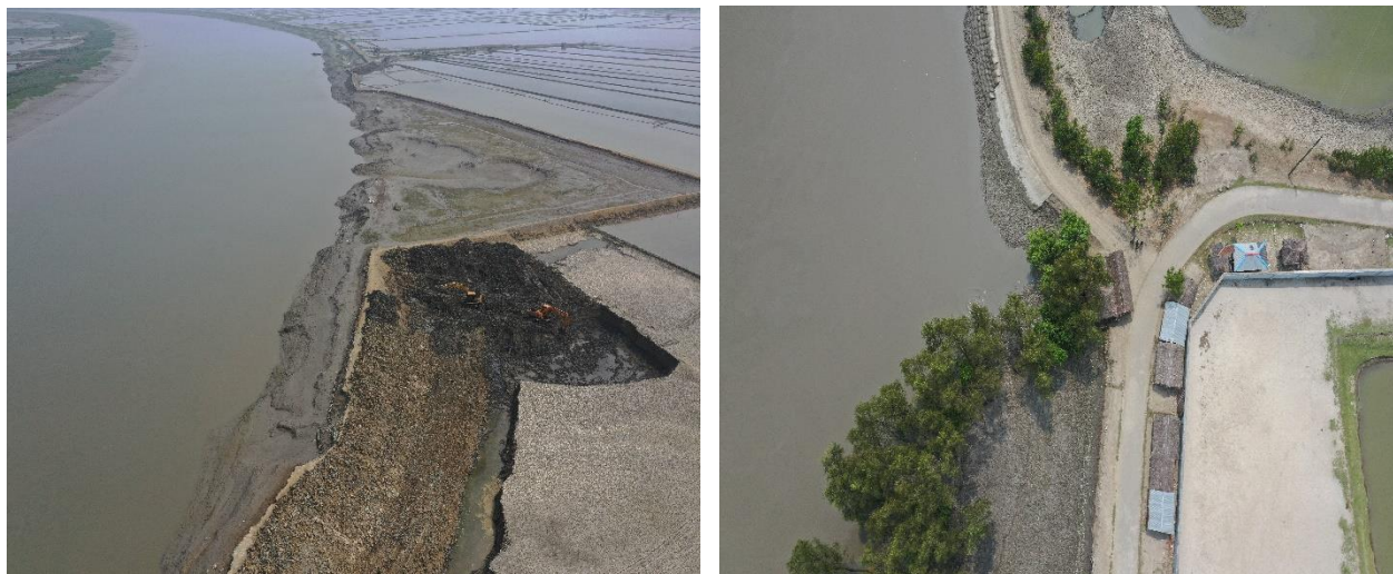
Figure 2-7: Existing Polder Roads of Polder 13_14/2
