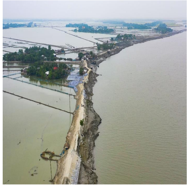
Figure 2-4: Damaged Polder 7/1 (Drone Survey View)
