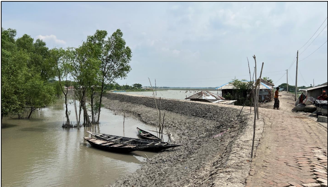
Figure 1-7: Koyra Polder 13-14/2 near Sundarban
