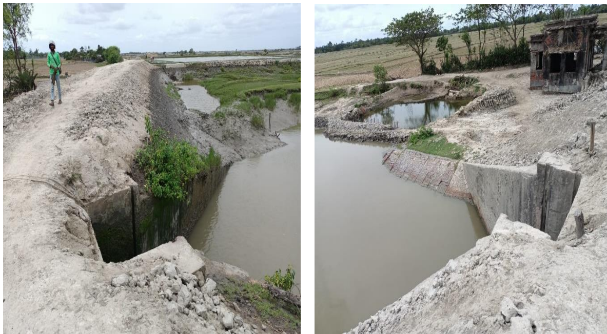
Figure 2-10: Existing conditions of the sluice gates in 7/2 polder
