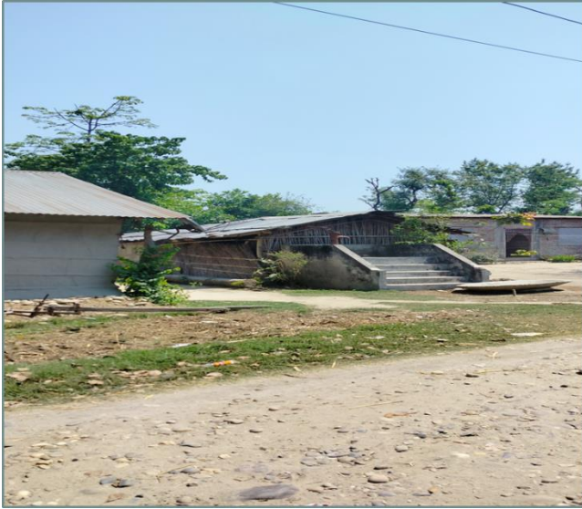
Elevated tube well
