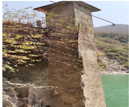
Photo 2: Flood Measuring Pillar in Rajapur
