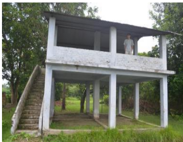
Concrete evacuation tower
