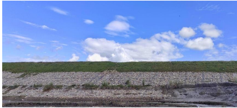
Figure 8: Riverside slope of the dyke
