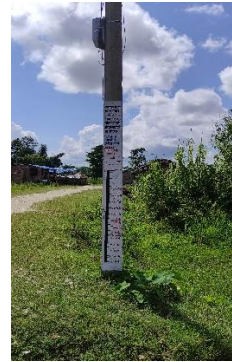
Electric pole with flood level measurement
