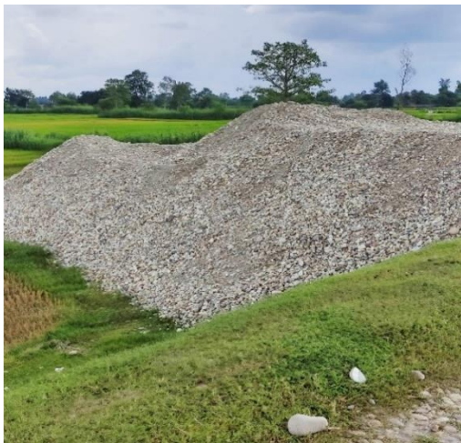
Figure 12: Materials for maintenance of dykes
