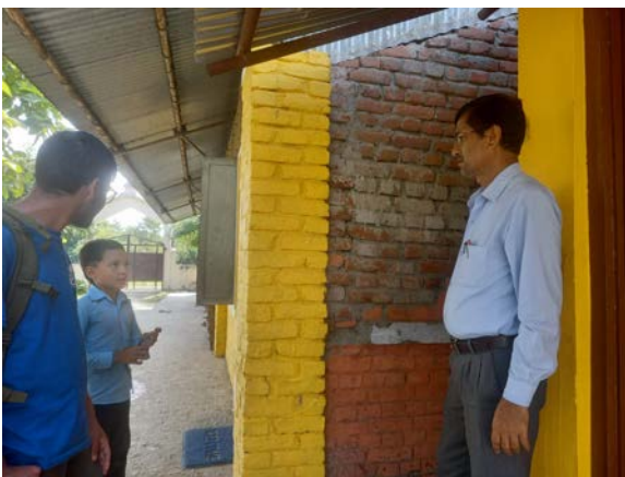
E. Reconstructed school building
