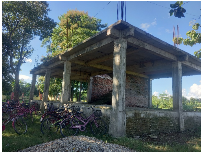
Figure 48: Ongoing construction of flood resilience school building
